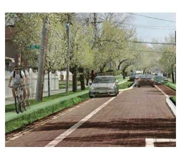
In Flushing, New York, a cloudburst street combines permeable pavement and green infrastructure to capture runoff.
