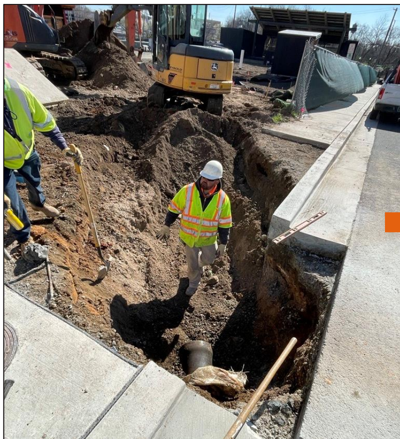
1: Pipe stub diverting offsite flow to park area
