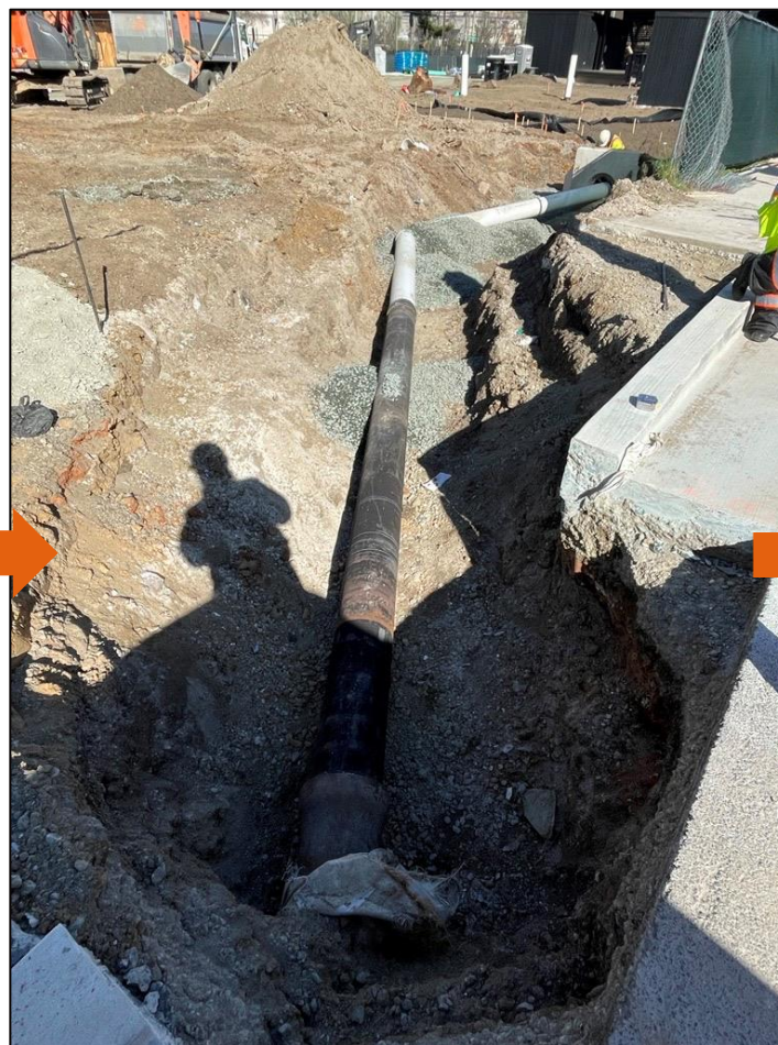
2: Pipe installation entering park area through rain garden 1 to headwall
