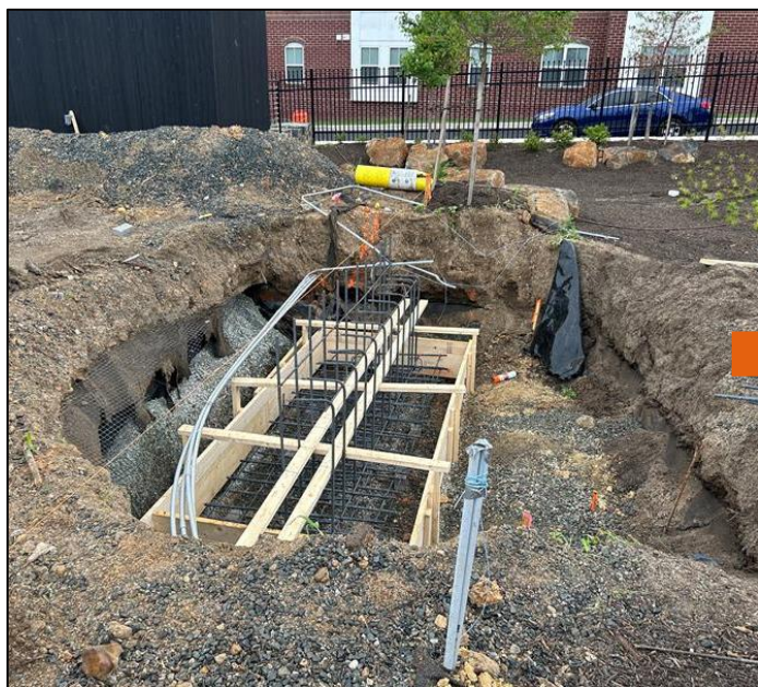
1: Installation of bridge & boardwalk foundations
