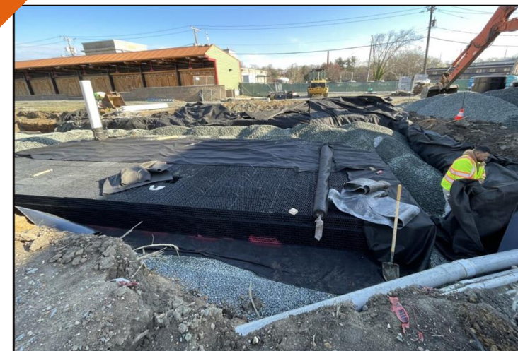
3: Installation of R-tanks
