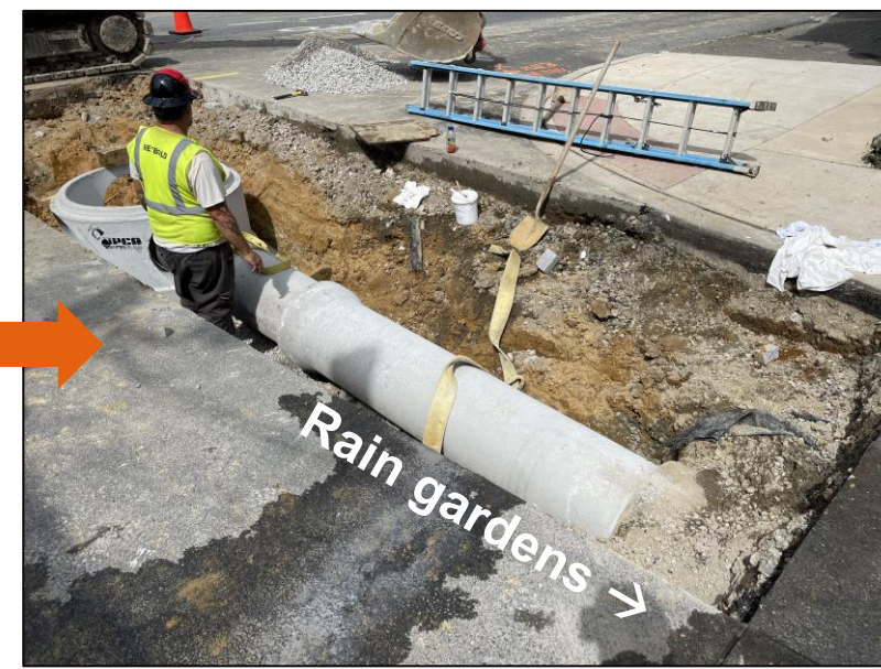
3: Storm sewer installation to connect these inlets to the existing pipe stub entering park.
