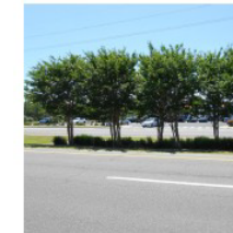
Figure 30: Route 1 Bioswales Trees are planted along one of the Route 1 Bioswales to help filter stormwater runoff and stabilize the facility.
