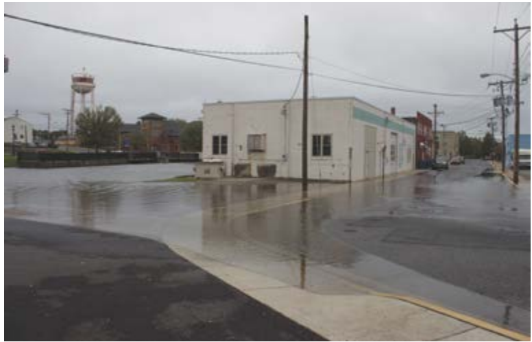
A nor'easter in October 2015 caused tidal flooding throughout the state. In Milford, the Mispillion River overtopped its banks, flooding business and roads adjacent to the river.
