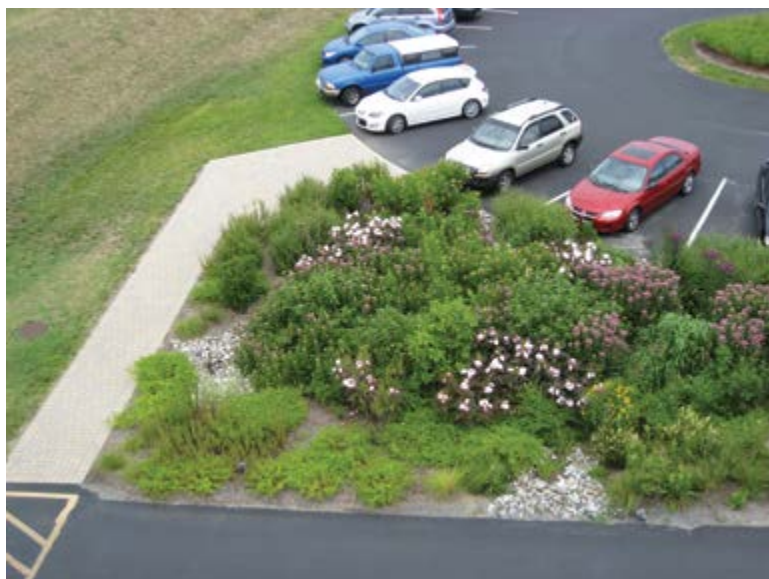
This rain garden at the Lewes Campus of the University of Delaware is a nature-based method to collect and store stormwater runoff from the parking lot that also provides habitat for pollinators and birds.
