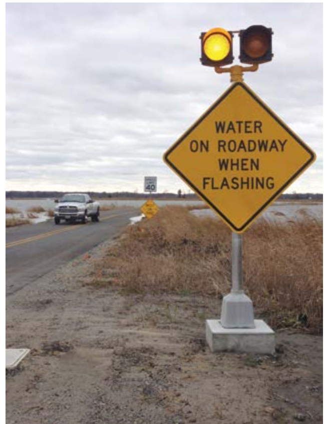
A permanent sign has been installed in the Primehook community in Sussex County to warn residents and visitors when the road may be impassable due to flooding. Credit: Susan Love, DNREC
